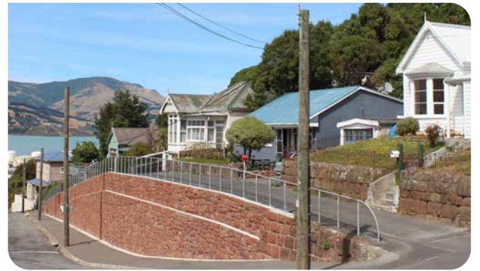
Reconstructed stone retaining walls, early 20th century houses
