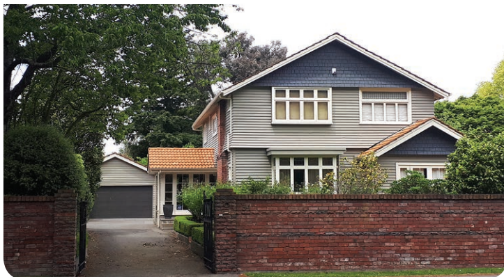
Weatherboard cladding, box windows, and shingle gable ends illustrated are characteristic features of English Domestic Revival
