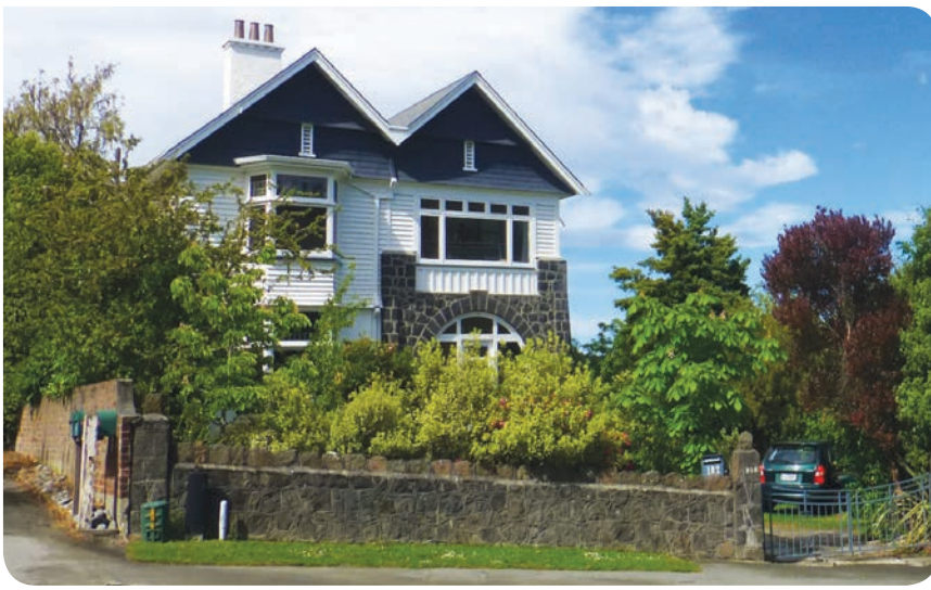
Example of English Domestic Revival Houses on Hackthorne Road
