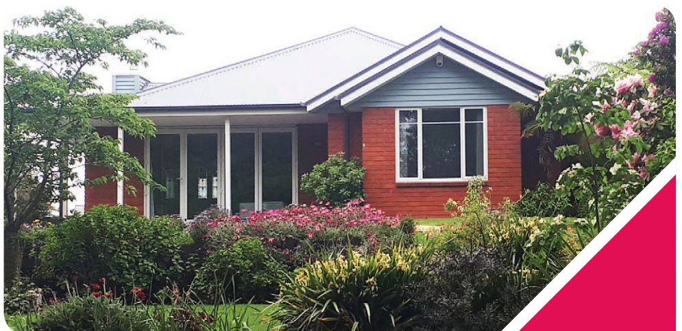
Contemporary brick bungalow with characteristic design features such as weatherboard gable ends
