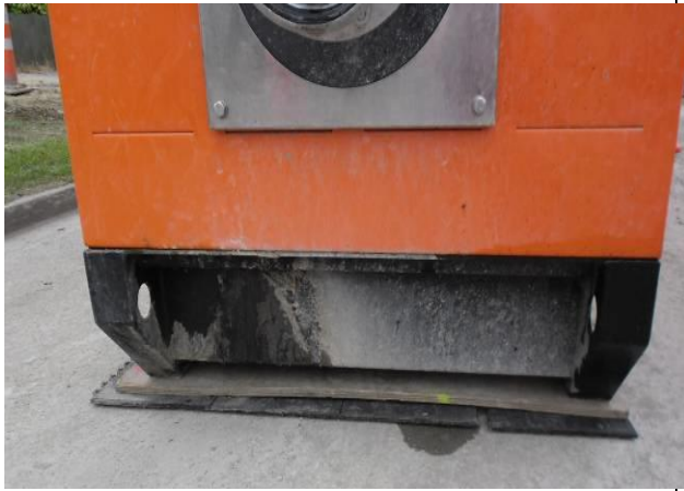
Figure 33: Noise Mitigation: Foam Mat and Plywood (to stop compression of foam)
