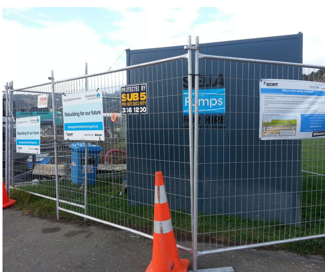
Figure 16: Locked site fencing around pump
