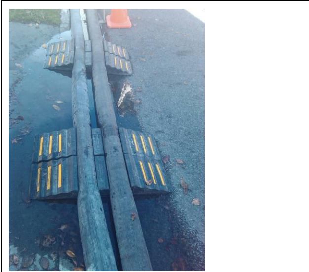
Figure 39: Pipe Protection: Ramps in front driveways
