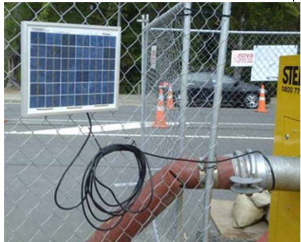
Figure 21: Solar Panel for Float Alarm
