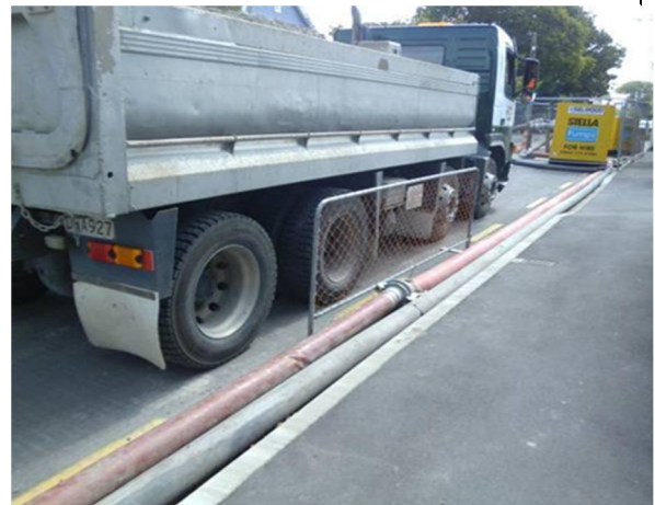
Figure 11: Traffic protection for pipes
