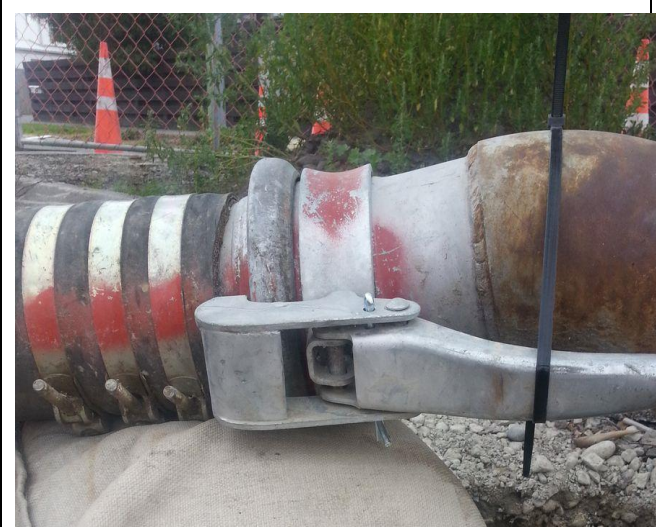
Figure 8: Layflat Pipe: Couplings secured
