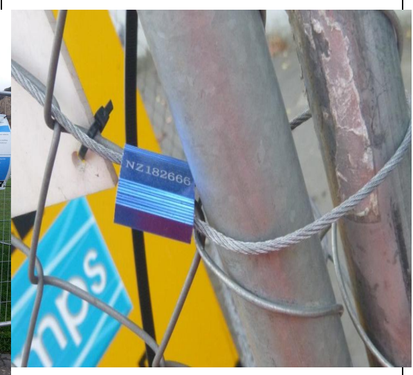
Figure 17: Wire ties to secure fence panels
