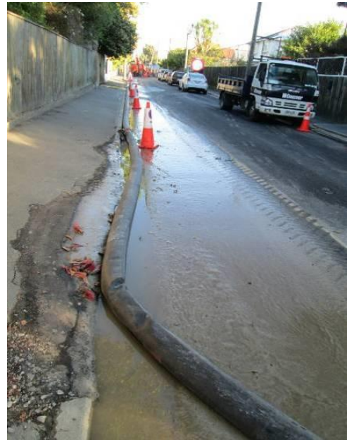
Picture 2: Wastewater sludge on a street following an overflow.
