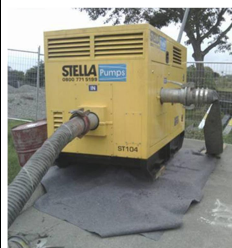
Figure 31: Spill Mitigation: X TEX Fabric under pump
