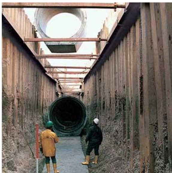
Figure 2-10 Sheet Piled Trench
