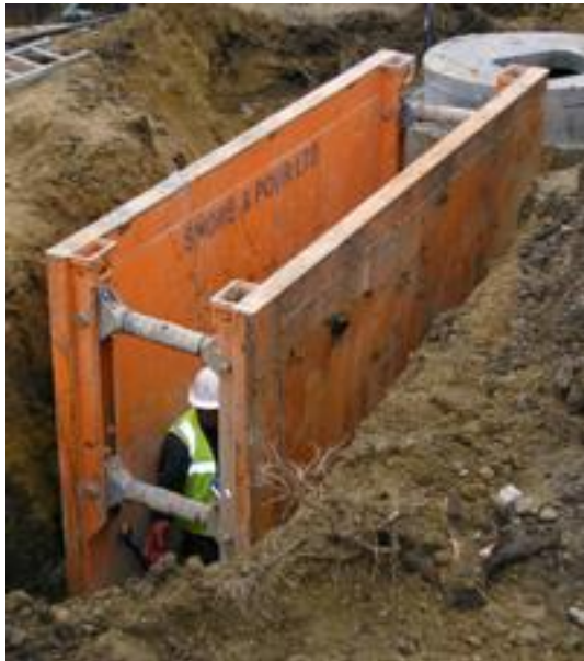
Figure 2-3 Shields protect workers but they do not necessarily support the trench walls
