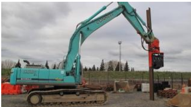
Figure 2-9 Installing Sheet Piles
