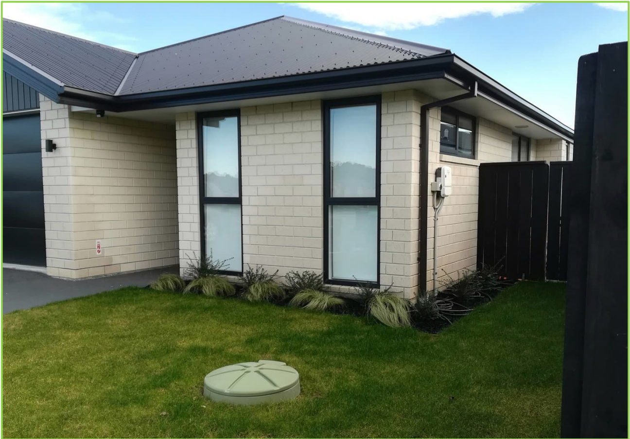
Figure 5 –Pump chamber completed installation position
