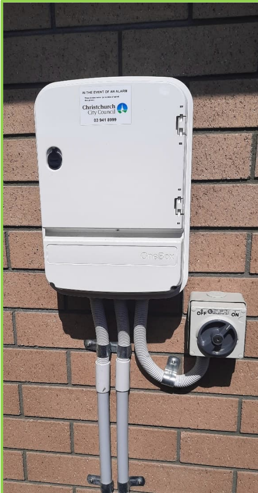
Figure 6 – Control panel completed installation position
