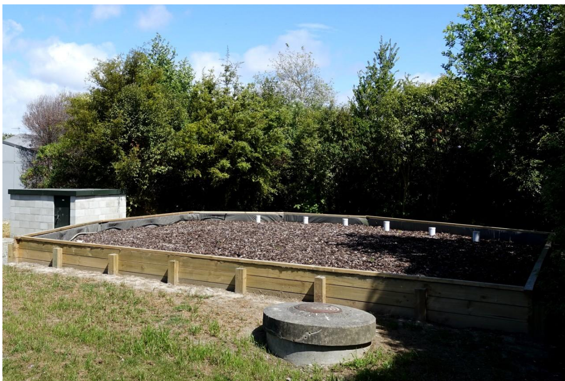
Photo: Pumping Station 11 Biofilter Randolph St - Station ID OC0477. Timber edging with media mostly below ground level.
