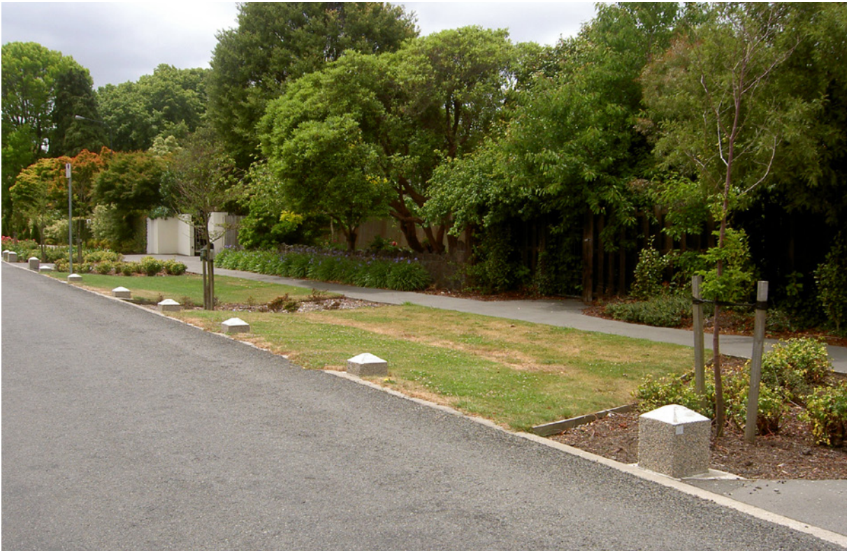
Bollards prevent vehicles parking in the swale (Waiwetu St)
