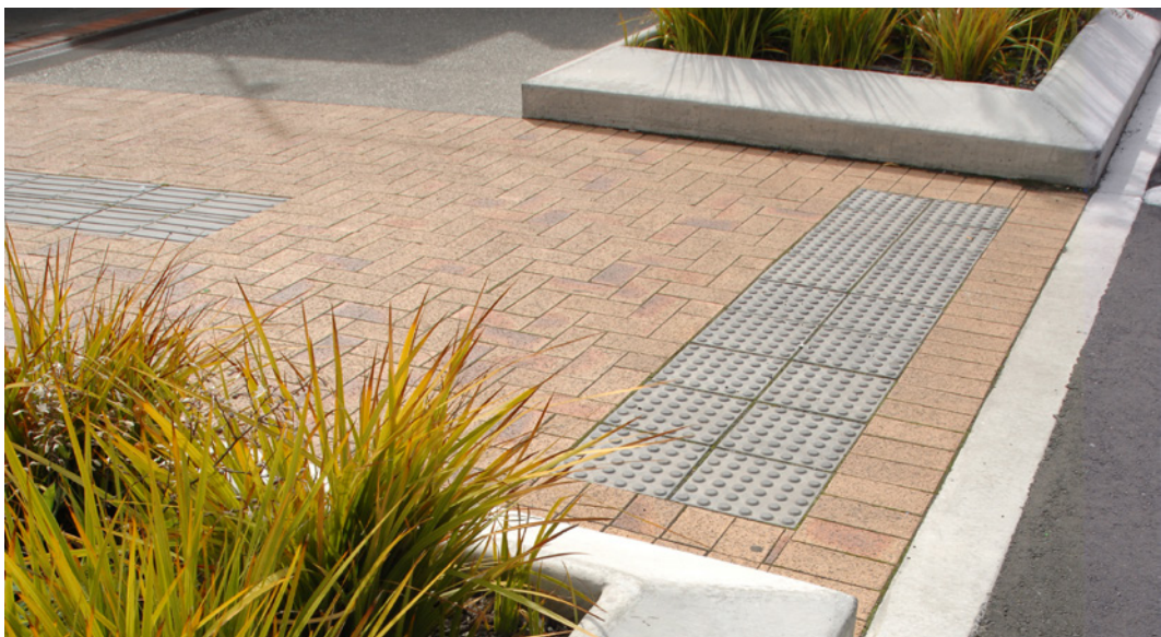
Tactile pavers at a pedestrian crossing cut-down (New Brighton Mall)
