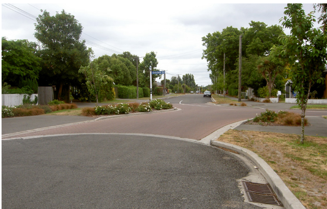
Reducing traffic speed through traffic calming (Geraldine/Gresford intersection)
