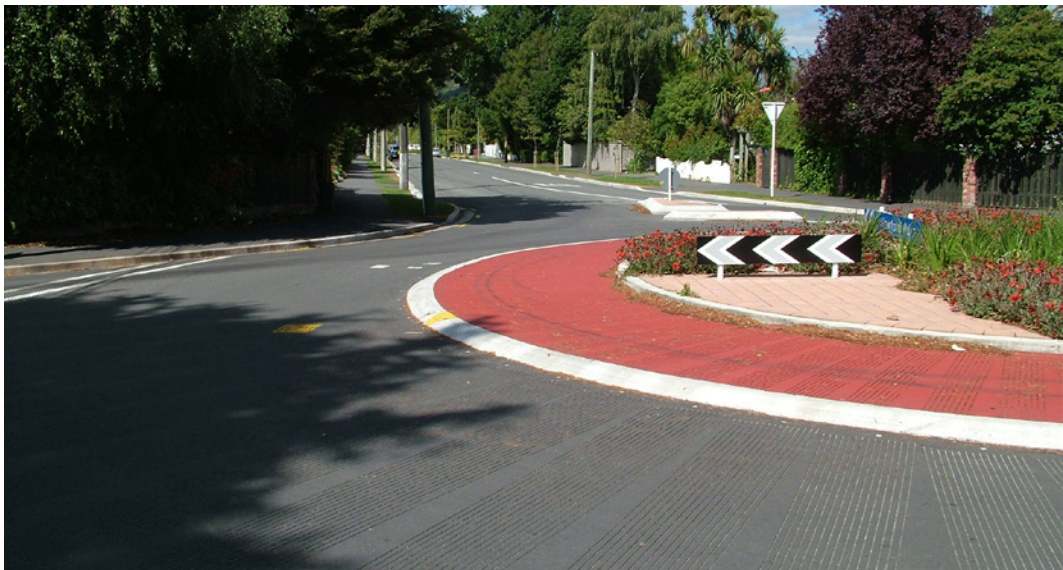
Roundabout with mountable apron (Hawford/Ford intersection)
