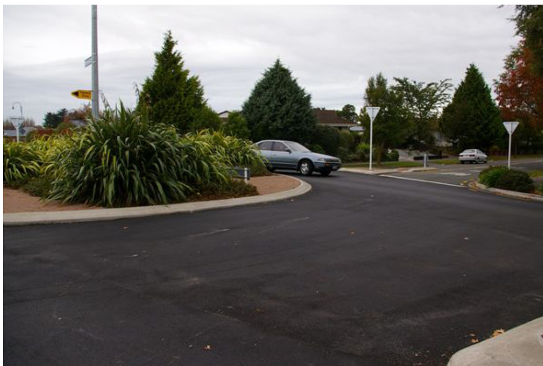
Planting that obstructs the visibility of approaching traffic
