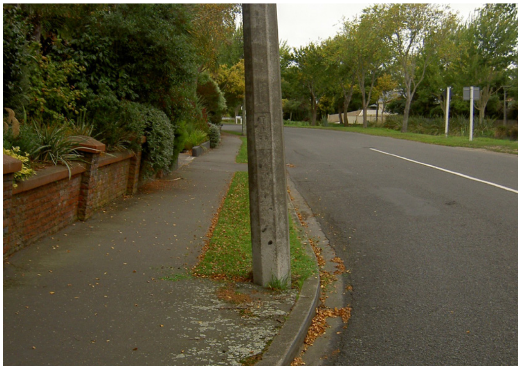
Squaring the point of a berm (Richardson Tce)
