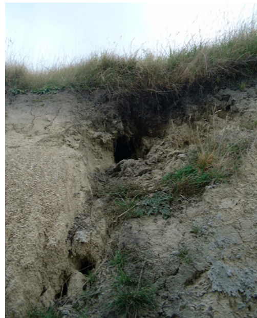
Tunnel gully exposed by earthworks
