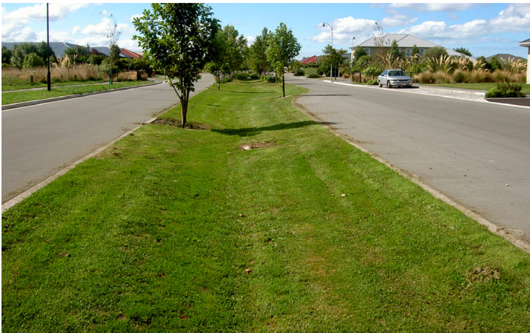
Temporary stormwater retention swale (William Brittan Ave)
