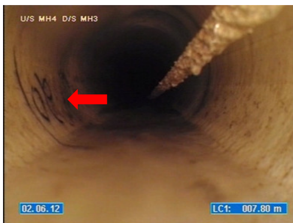
Photo, left, shows notes marked on the liner during wet out.
