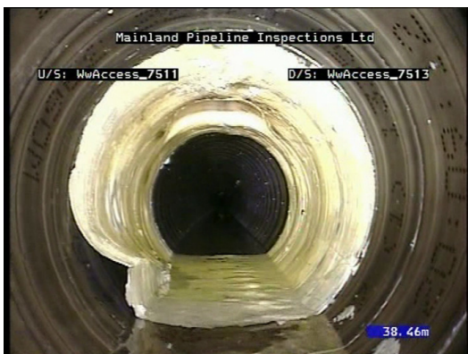
Medium PL, LJR/LCR lifted/separated from the spiral wound liner.
