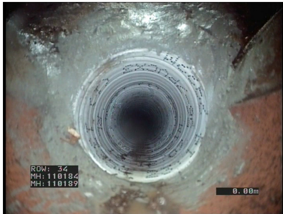
Good example of an end seal and transition in an Expanda (Spiral Wound) pipe.
