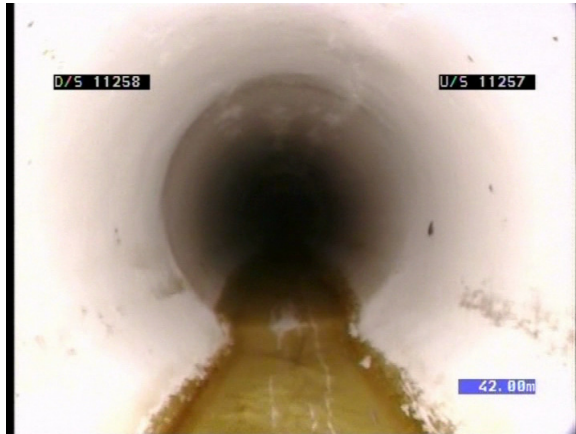
Flexible liner showing reflective shape of the pipe beneath the liner.
