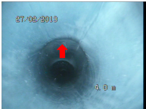
Flexible liner, above, installed in a deformed lateral junction – liner takes on the deformed pipe shape.
