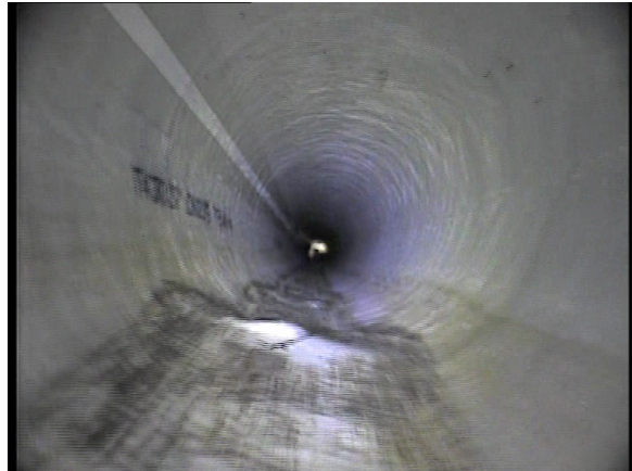
Small, bulge in the liner, appears that there was debris in the pipe, not removed, prior to lining
