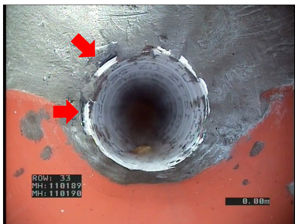
Good example of an end seal and transition in an Expanda (Spiral Wound) pipe.
