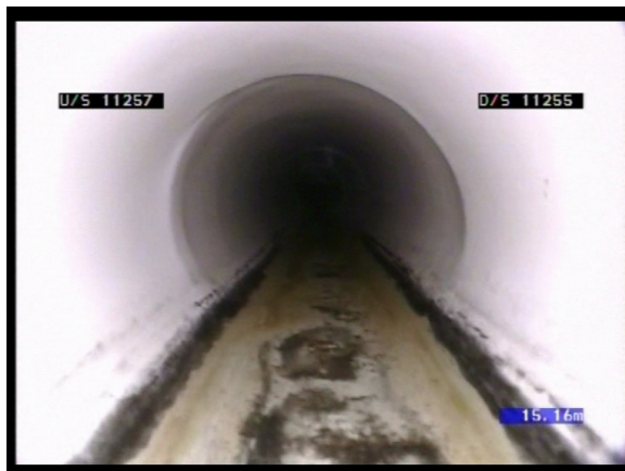
Another example, above, of a flexible liner over a displaced joint in the host pipe
