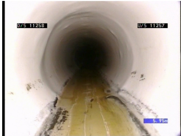
Flexible liner over a minor displaced & open joint in the host pipe
