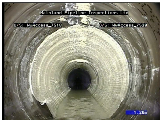
Small, bulge where the liner has gone over an object.
