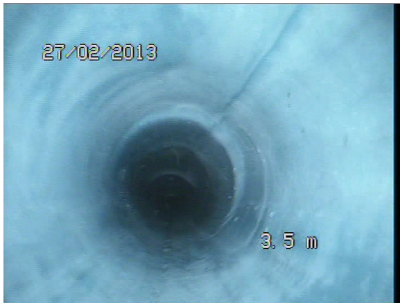
Flexible liner over what appears to be either a slight displacement or an uneven (irregular) wall thickness at the joint that you commonly see in EW pipes.
