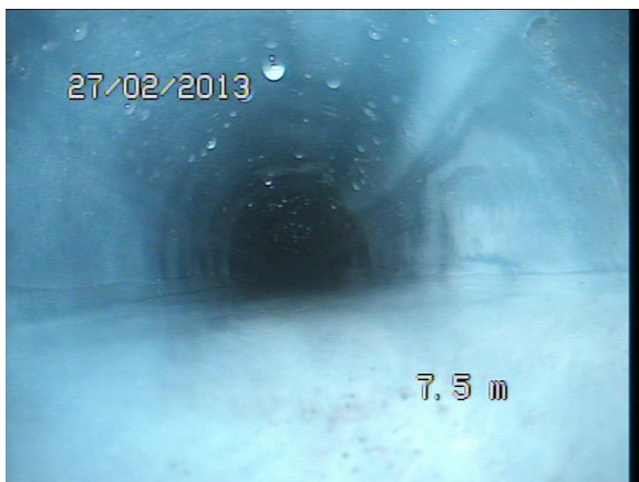
Flexible liner over what appears to be either a slight displacement or an uneven (irregular) wall thickness at the joint that you commonly see in EW pipes.
