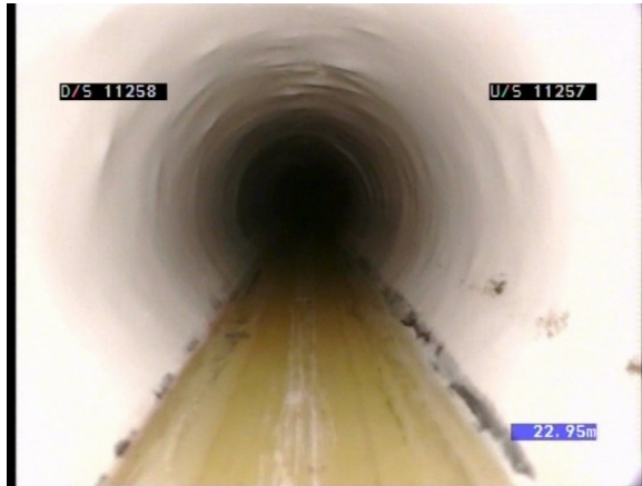
Flexible liner showing reflective shape of the pipe beneath the liner.
