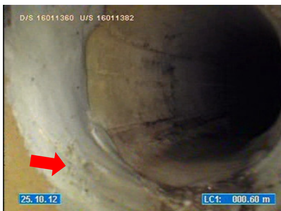
Good transition, but the end seal has gaps between the Expanda liner and the host pipe – Gap, but no evidence of pathway, coded as JF, Medium.
