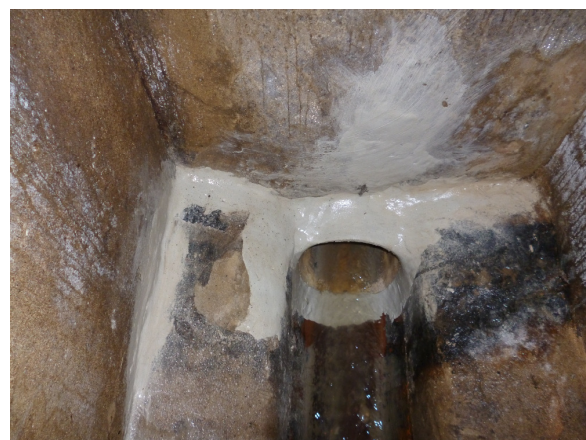
Excess mortar on the end seal causing rough entry and an obstruction – coded as OP, Small.
