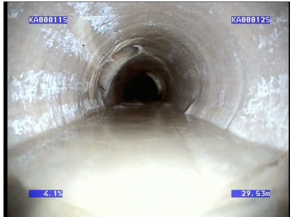
Flexible liner over a minor displaced & open joint in the host pipe
