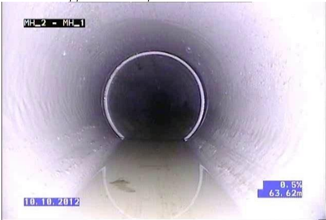
Photo 3: 300mm pipe with a 20 mm Dip
