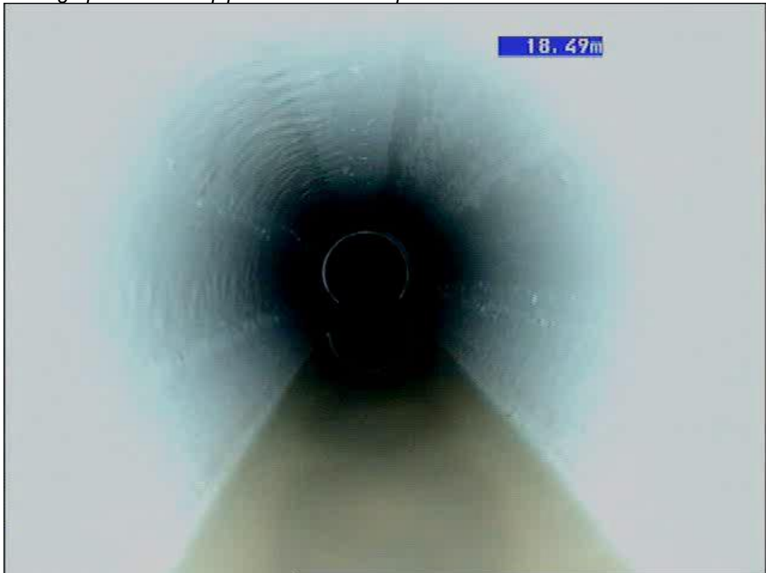
Photograph 1: 150mm pipe with a 20mm Dip
