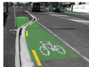
Figure 3 – An example of a cycle lane denoted by the NZTA approved cycle lane symbol
