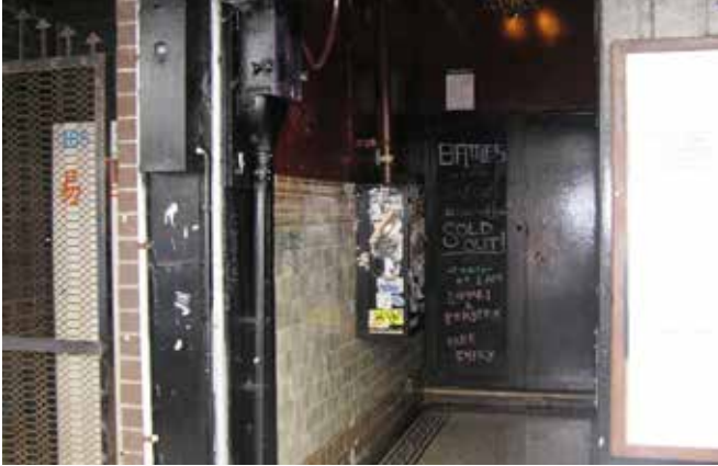
Example of poor entranceway to a nightclub
