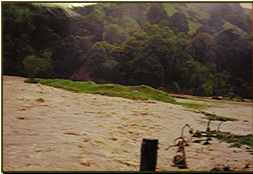
Stream torrent over stop bank. Fallen willows on far right.
